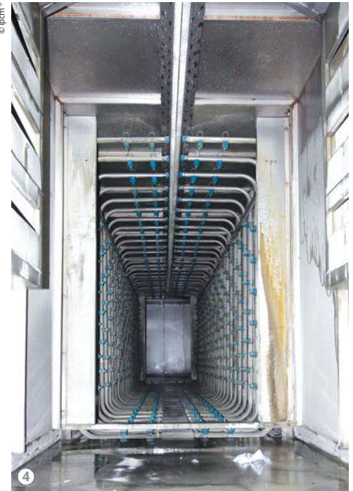
Figure 4: The pre-treatment tunnel
