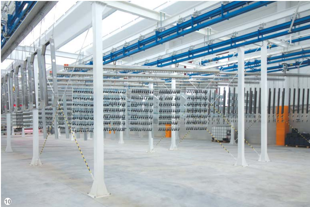
Figure 10: Futura Convogliatori's two-rail conveyor.
